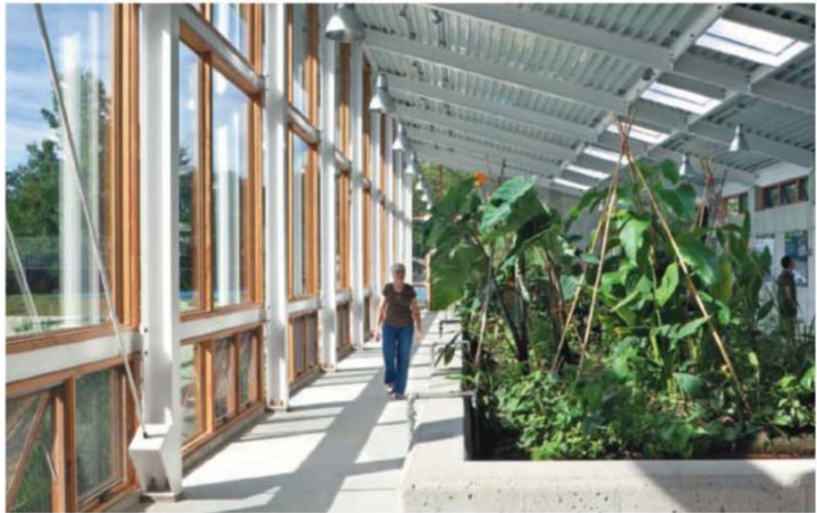
Above The OCSL has a greenhouse-like atmosphere with solar-tracking skylights and south-facing glazing providing the daylight that the Eco-Machine's water-scrubbing plants need to thrive.
