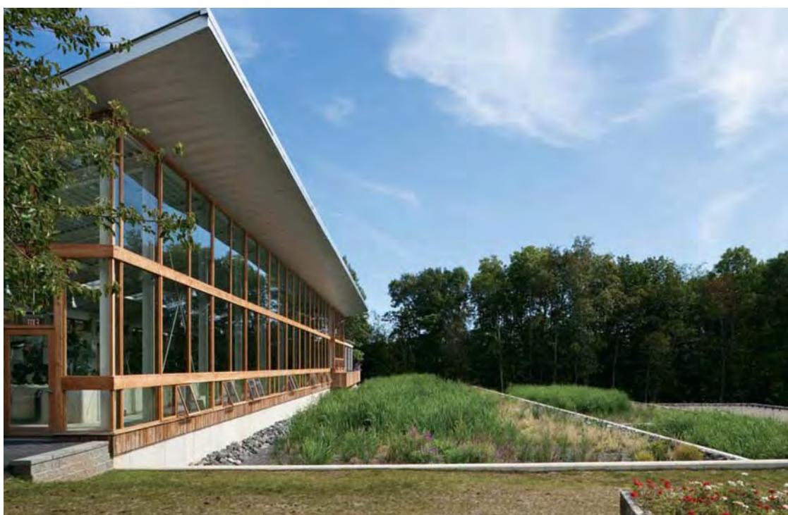
Above Four distinct cells make up the outdoor constructed wetlands, just south of the building. Campus wastewater enters these wetlands early in the cleansing process. This nutrient-rich water ensures a robust landscape for the southern view from the building.
